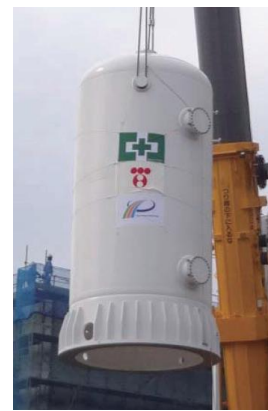
Filtered Venting Vessel for the Kashiwazaki-Kariwa Nuclear Power Station (developed in-house)
